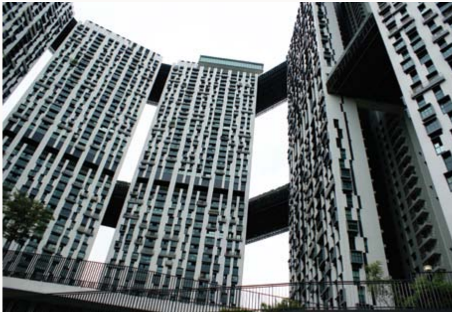
In an effort to create more environmentally conscious public housing, HDB has begun offering innovative housing projects such as the Pinnacle@Duxton. The development integrates private living and public communal spaces in high-rise, high-density living, and was designed to enhance energy efficiency by maximising natural airflow and light and minimising sun exposure. Pinnacle@Duxton, 2012. Courtesy of Joanna HS Tan.
